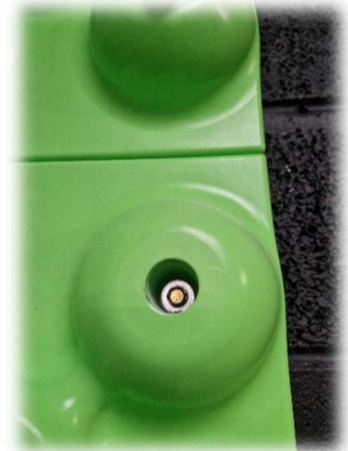
Use minimum 6 fixing points
